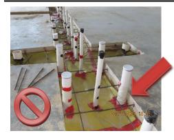
When the slab cut is made, make sure that at least 6" of room adjacent to any pipe penetration.
